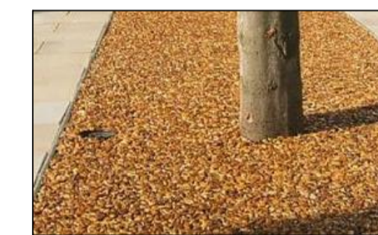
STEEL FRAME (RESIN BOUND INFILL)
